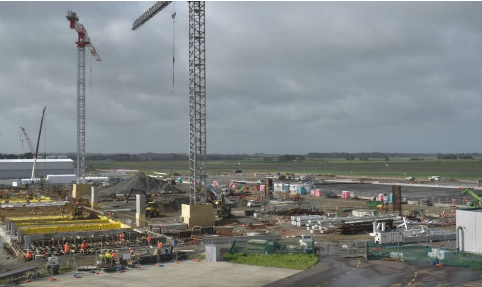
Left: groundworks at RNZAF Base Ohakea.
